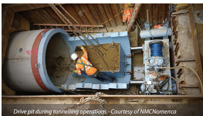
TBM launch - Courtesy of NMCNomenca
