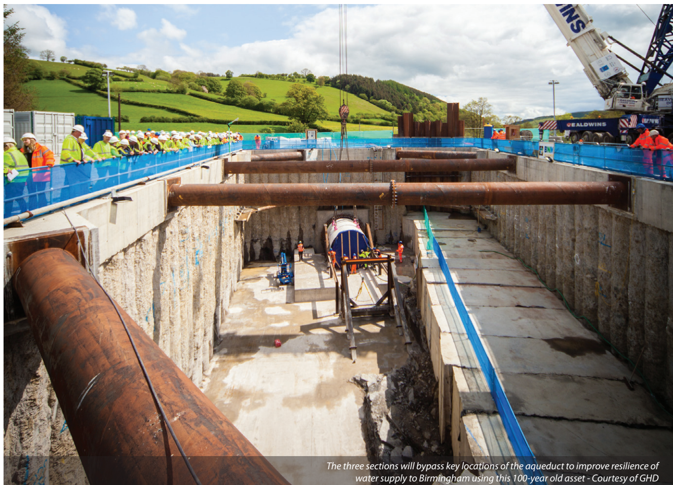
BNMA's design meant the flows could be turned in to the new bypass section without shutting the aqueduct down
