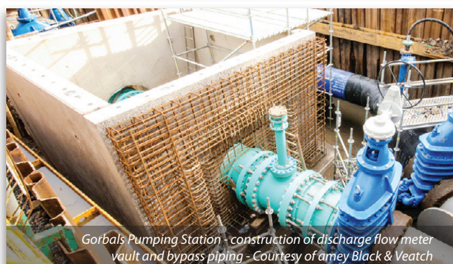
Gorbals DSR - construction of new valve station Courtesy of amey Black & Veatch
