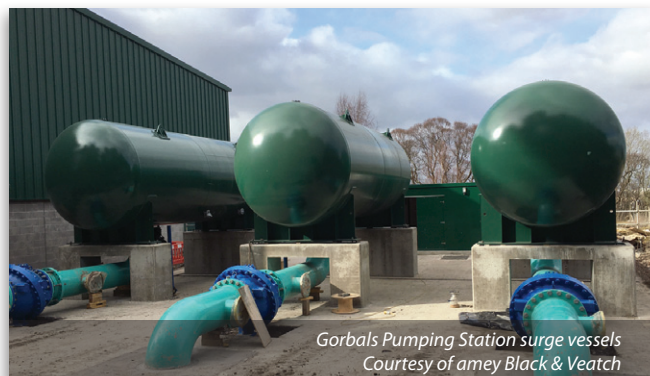
Gorbals Pumping Station - exterior view showing surge vessels Courtesy of amey Black & Veatch
