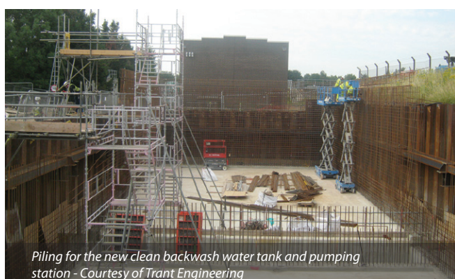
Construction of 8 (No.) GAC filters - 4 (No.) filters either side of a central gallery - Courtesy of Trant Engineering
