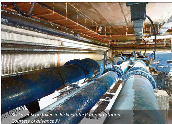
The existing water pipes are being replaced with new larger pipes under the project scope - Courtesy of advance JV
