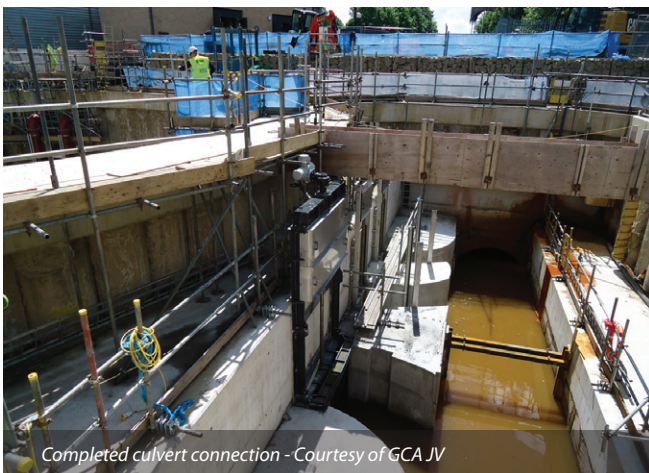
Partial culvert connection - Courtesy of GCA JV
