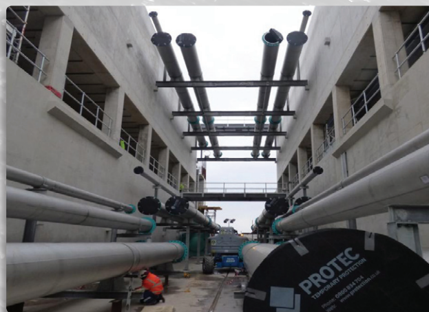
Central gallery under construction (DfMA) - Courtesy of United Utilities
