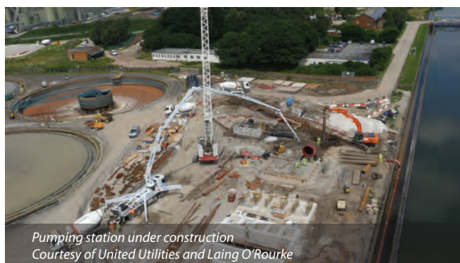
New inlet works under construction Courtesy of United Utilities and Laing O'Rourke
