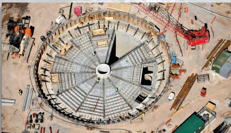
Precast roof install Courtesy of C2V+
