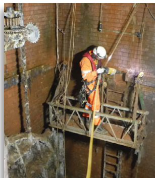
Confined space structural repair
