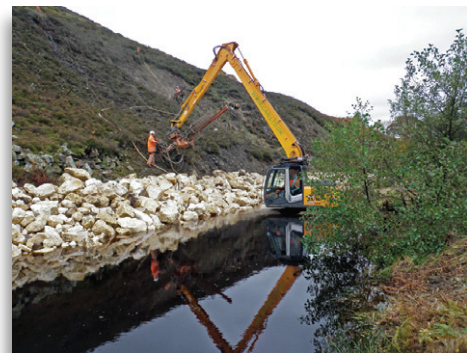
Soil nailing and netting to safeguard assets
