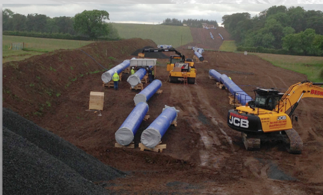
Excavation prior to pipe laying Courtesy of Caledonia Water Alliance
