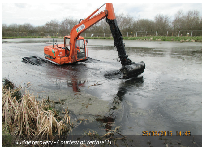
Sludge agitation and recovery - Courtesy of VertaseFLI
