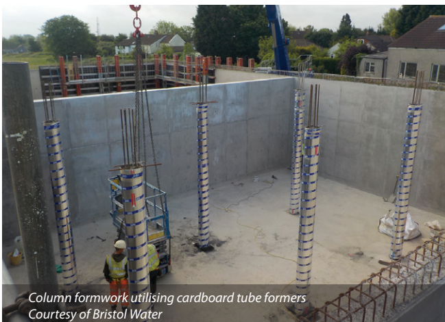
Original reservoir site following decommissioning and construction of the communication tower base slab (utilising one compartment of the old reservoir) - Courtesy of Bristol Water
