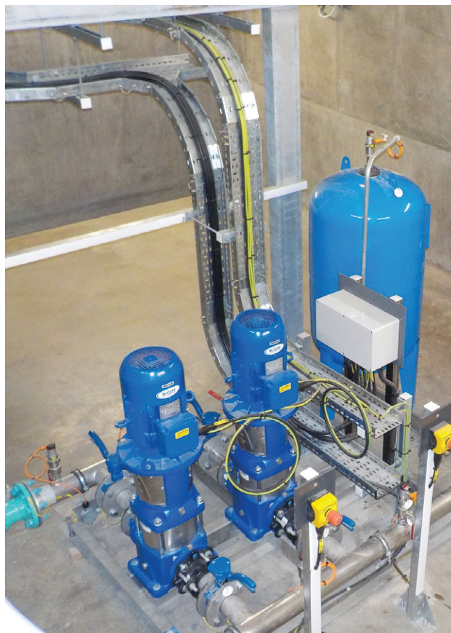
Skid mounted package pumpset including hydropneumatic vessel Courtesy of Bristol Water
