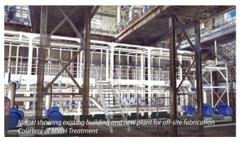
To address many of the existing issues at source the new lime plant arrangement is able to use the latest technology to consistently produce a dissolved limewater solution (0.13% w/w) rather than a lime slurry.
