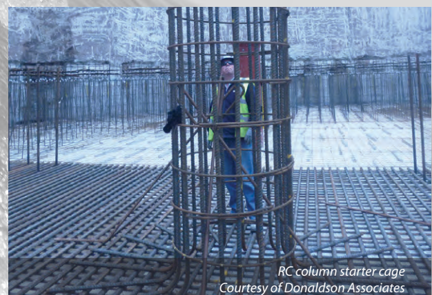
Fixing of the Sheargrid on site - Courtesy of Donaldson Associates
