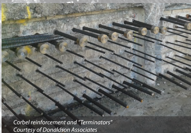
Installation of threaded bars - Courtesy of Donaldson Associates
