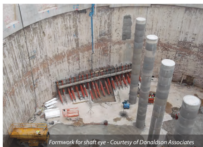
Base slab showing the rebate and columns Courtesy of Donaldson Associates
