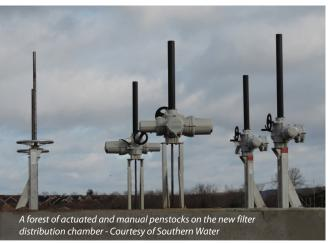
minimum of structural modifications. A means of by-pass in the event of more than one screen being unavailable was also built into the design by installing a new manually raked screen in a dedicated channel with its own actuated penstock.
