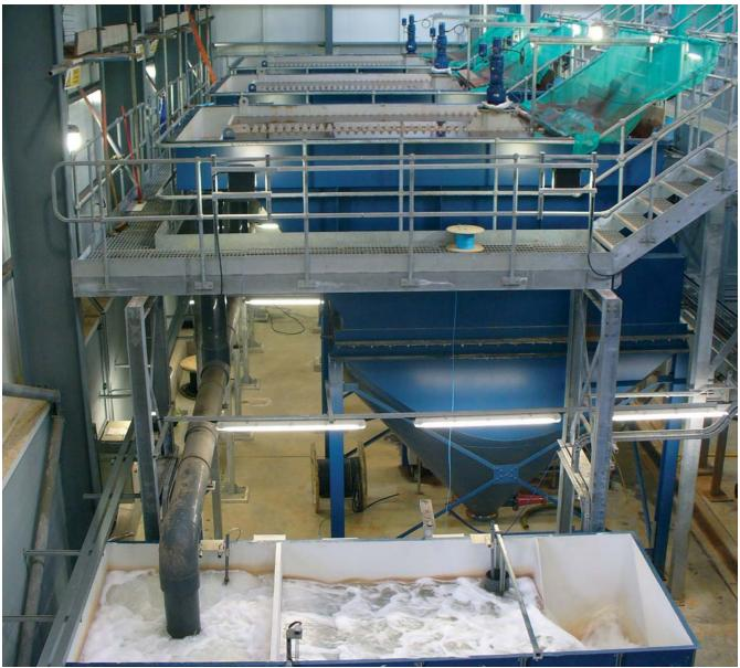
Clarifiers and final effluent chamber
