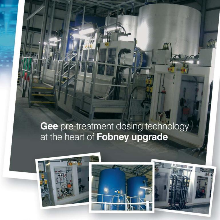
Under a contract awarded by Veolia Water Solutions and Technology (VWS), Gee & Company has installed the bulk of the dosing equipment for the Actiflo TM clarification process to treat abstracted water as part of Thames Water's upgrade of Fobney Advanced WTW in Reading.
