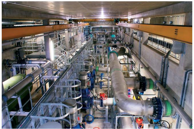
Douglas IOM WTW: Treated water pump gallery (with backwash & interstage pumps in background
