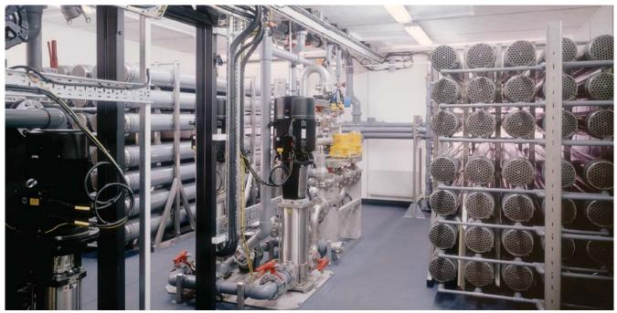
Interior of a Fyne Package Membrane Plant
