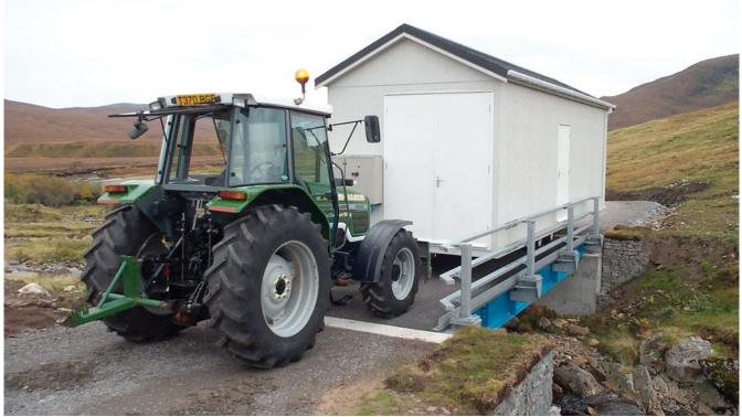
A Fyne Package membrane plant being delivered to a remote site
