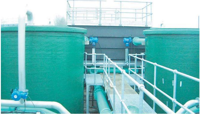
SAF tanks installed within clarifier structure - flow distribution tank in background
